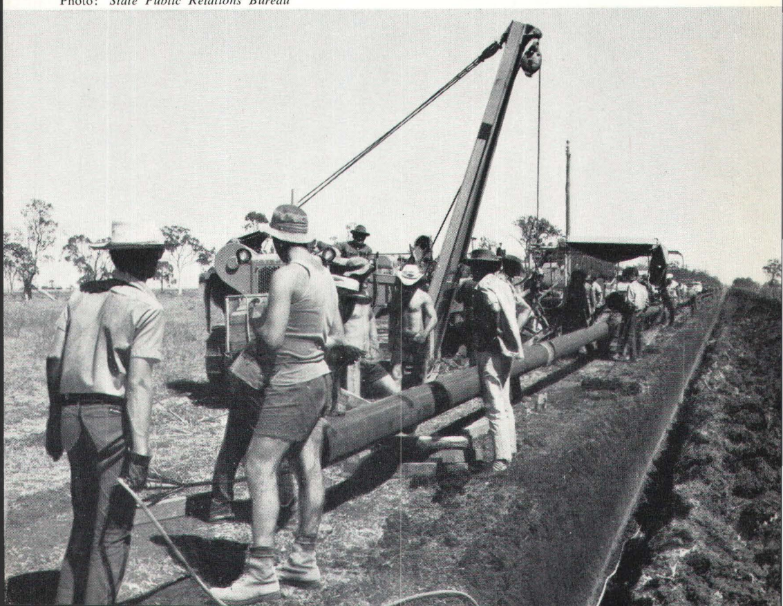
Laying of natural gas pipeline from Roma to Brisbane
